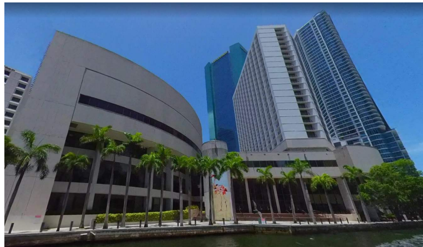
11. VIEW FROM SOUTHWEST MIAMI RIVER
