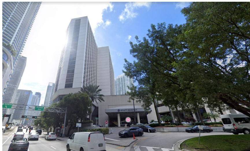
3. VIEW FROM NORTH SE 2nd AVE
